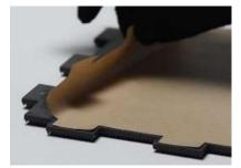
$\checkmark\,$  Position the tile to its final location and apply pressure perpendicularly across the surface with a flat palm /tool
